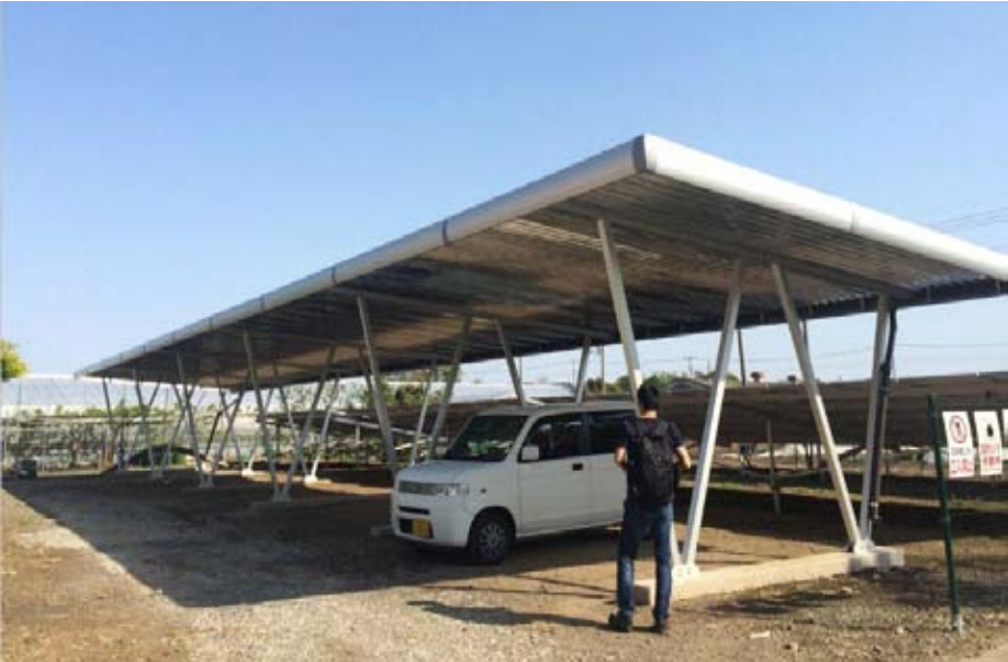
WATERPROOF CARPORT TOTAL LAYOUT: 10 Cars MATERIAL: Aluminium 6005 - T5
