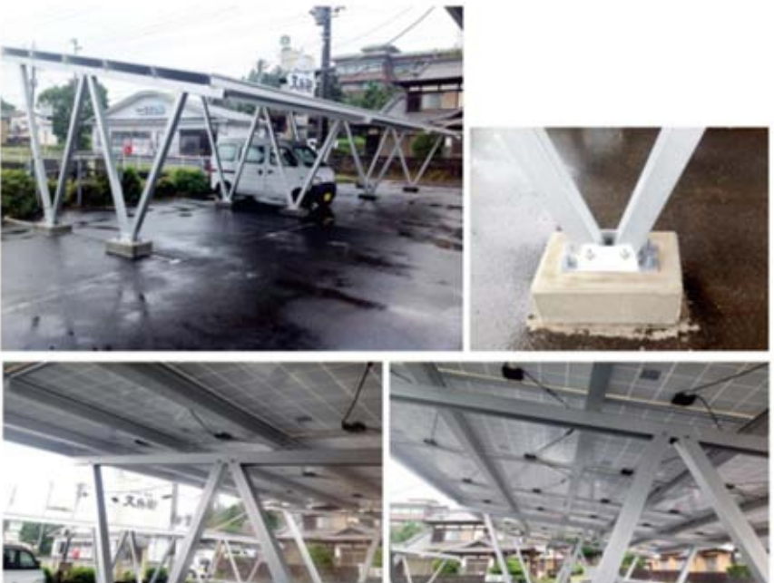
WATERPROOF CARPORT TOTAL LAYOUT: 6 Cars MATERIAL: Aluminium 6005 - T5
